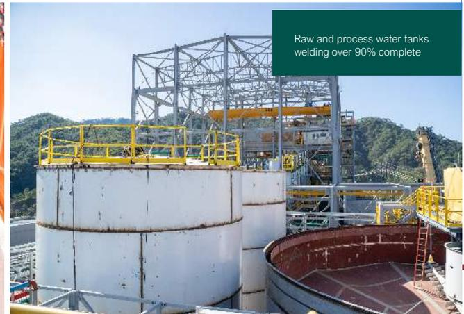
Raw and process water tanks welding over 90% complete
