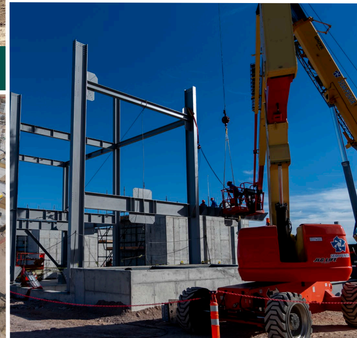
Mill platform structural steel
