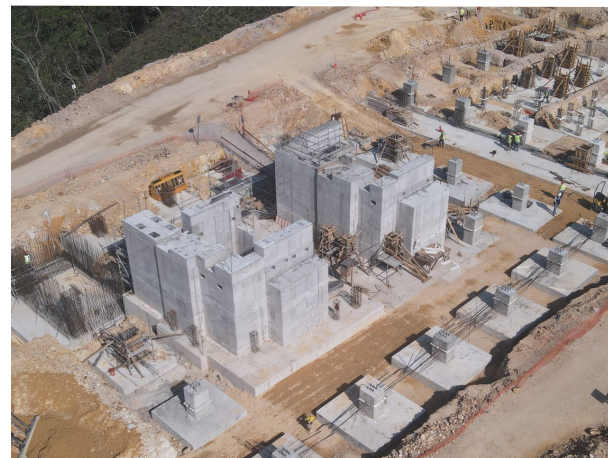
Grinding area ready for mechanical installation
