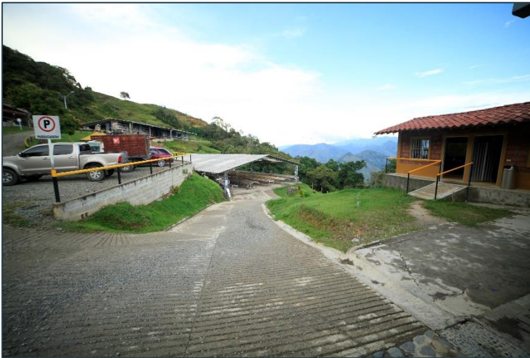
Titiribi Office and Core Facility
