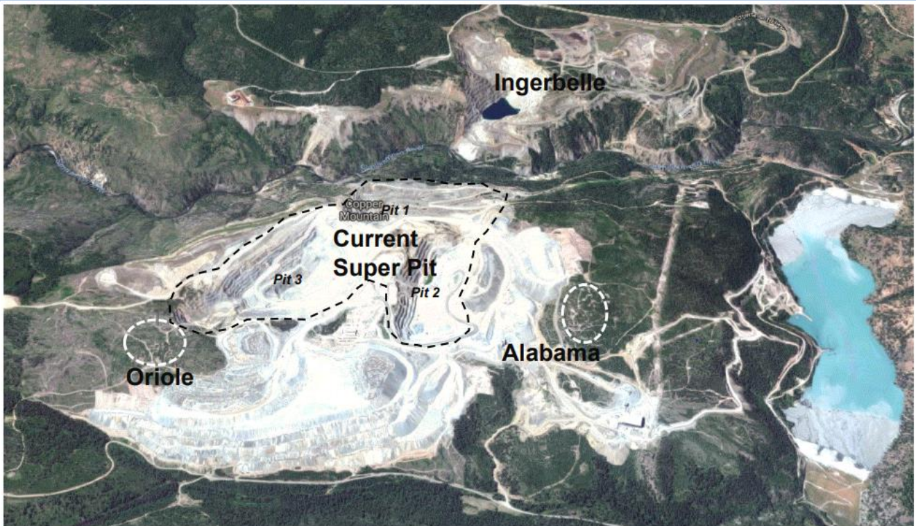
Fig. 3: Copper Mountain Mine Layout
