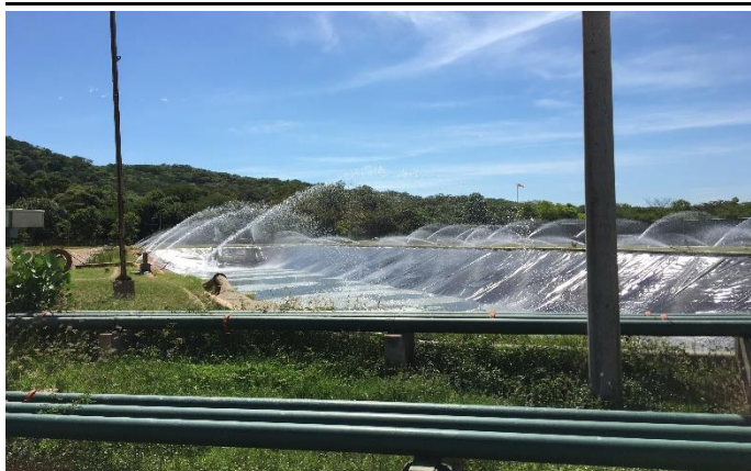
Figure 15: Cooling ponds
