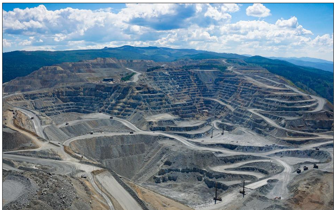
Figure 3: Copper Mountain Main Pit Panorama
