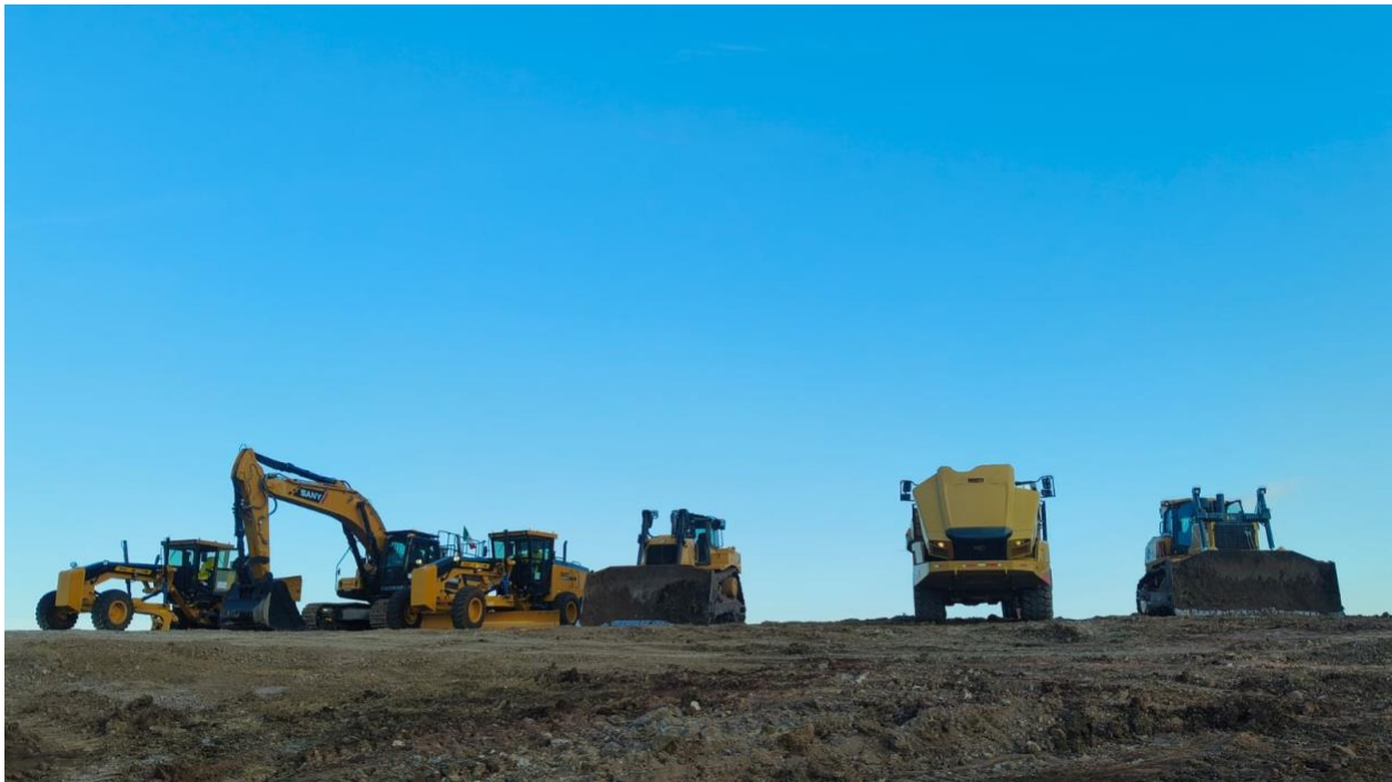
Figure 2 – Construction Equipment on Site
