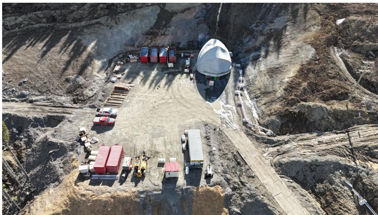
Figure 5: Lowhee Zone ventilation raise bore.
