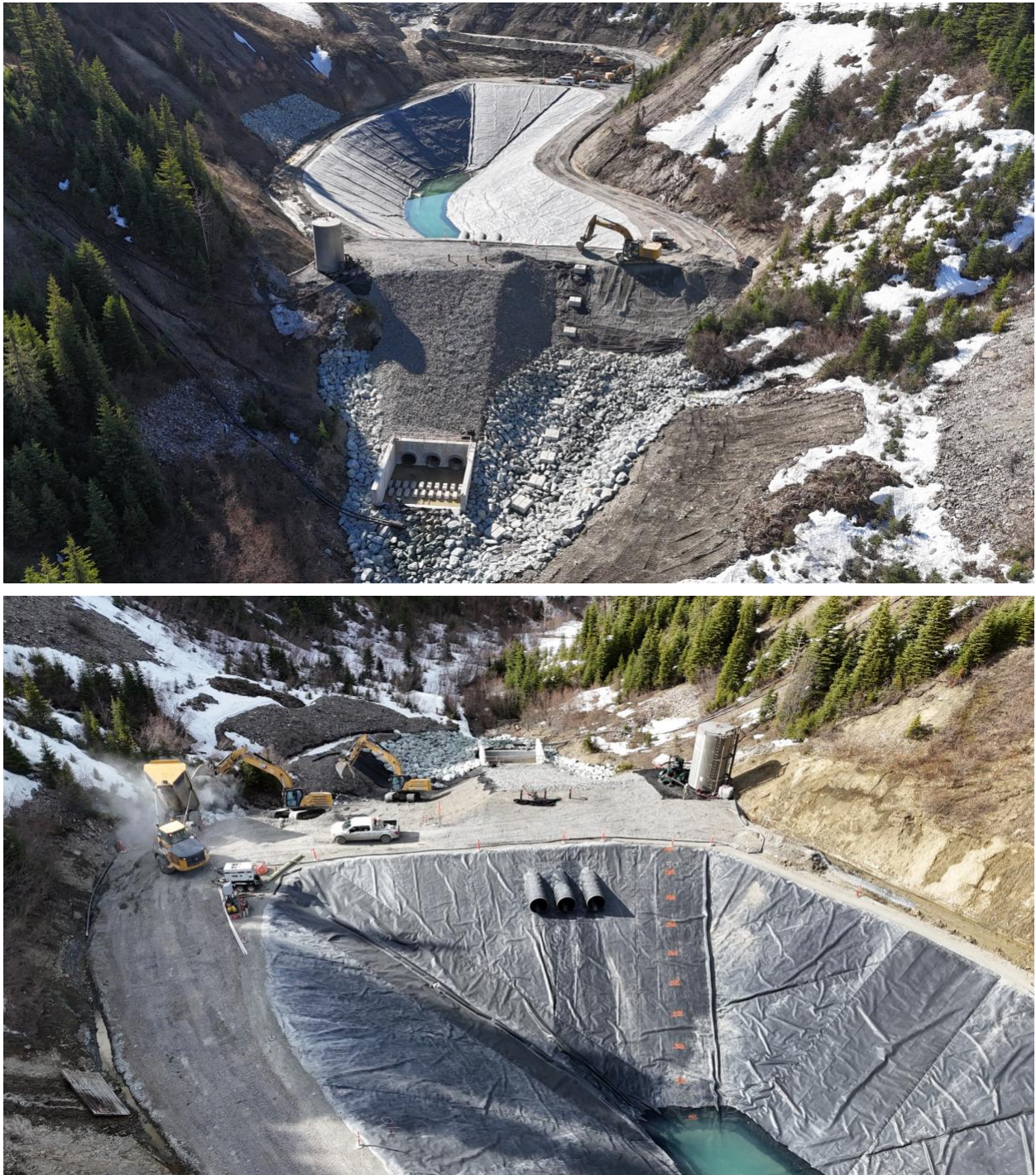
Figure 2: Sediment control pond (SCP) installed liner and placement of aggregates.
