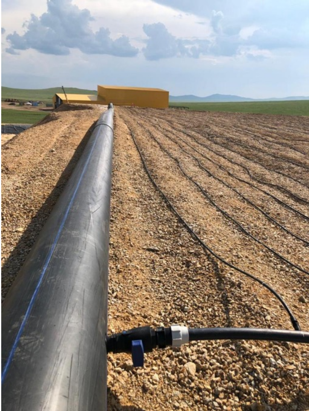
Main irrigation trunkline with the ADR plant in the background.
