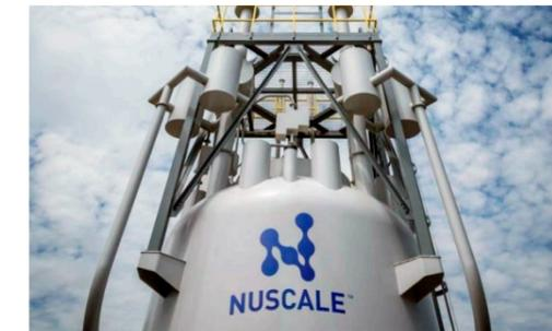
Demonstration model of a NuScale power supply module/small reactor.
